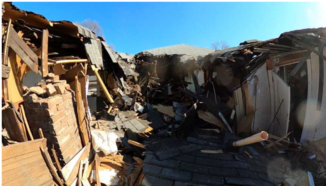
(1) Residential building collapse scene. Photos by Clinton Crafton.
