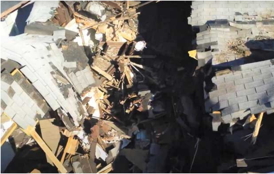
(2) Aerial view of collapse filmed using UAV.
